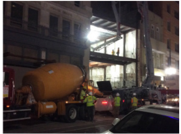
Early morning concrete pour for the 'gold building' which houses the hotel's restaurant.
