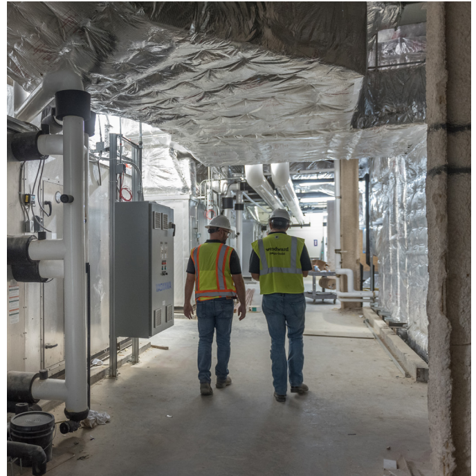
Project managers walk the site during construction
