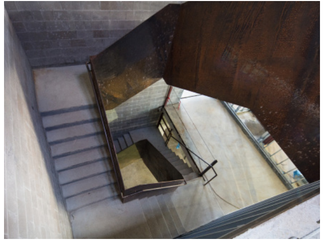
Steel and concrete staircase under construction
