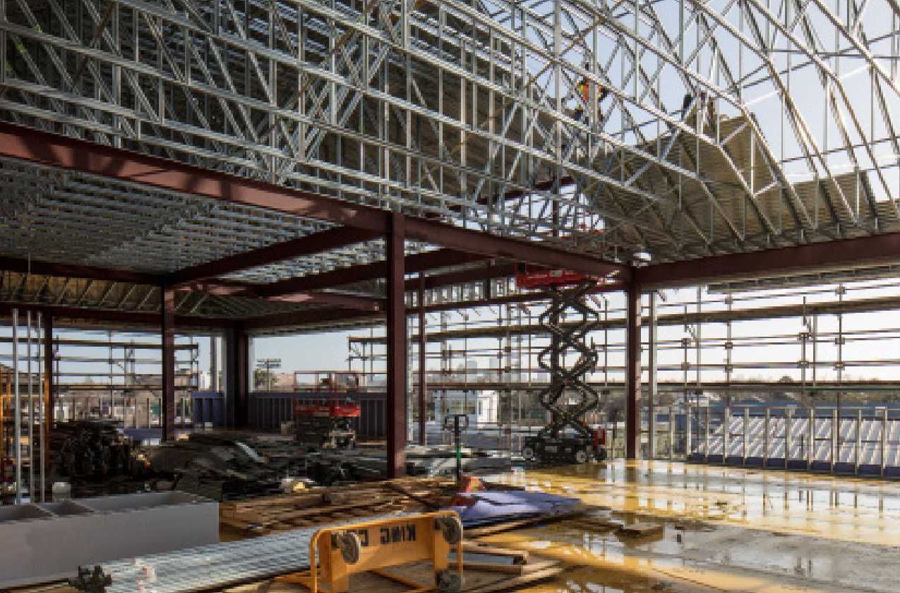
Second floor interior during construction
